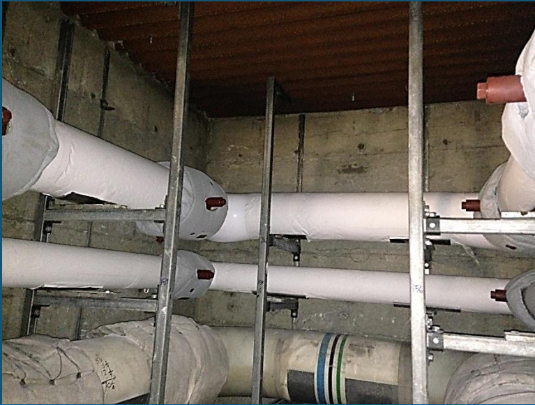
North Utility Tunnel Steam Pipe
