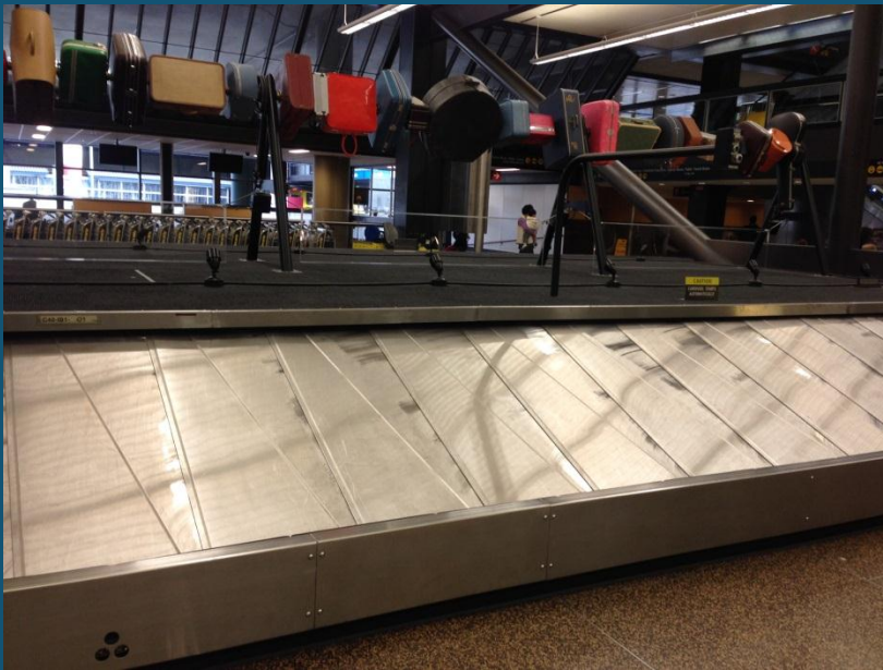
Refurbish Bag Claim Device
