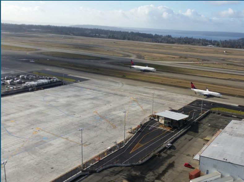
Aircraft Remain-Overnight facility
